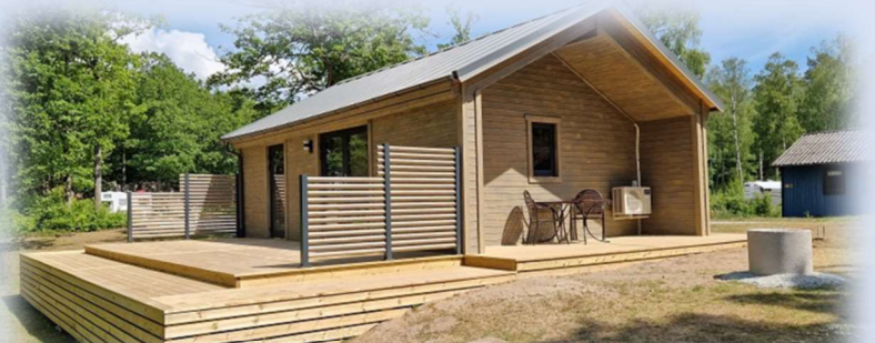
COTTAGE S13 AFTER RENOVATION
